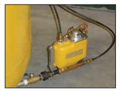
\* For operating pressures less than 60 psig, a source of pilot air of 60 to 225 psig must be supplied for cylinder operation. Viton and Teflon are registered trademarks of DuPont Corporation.
